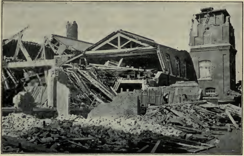
FIG. 599.— This building was torn in pieces by the shaking of the earth during one of the destructive Japanese earthquakes.
